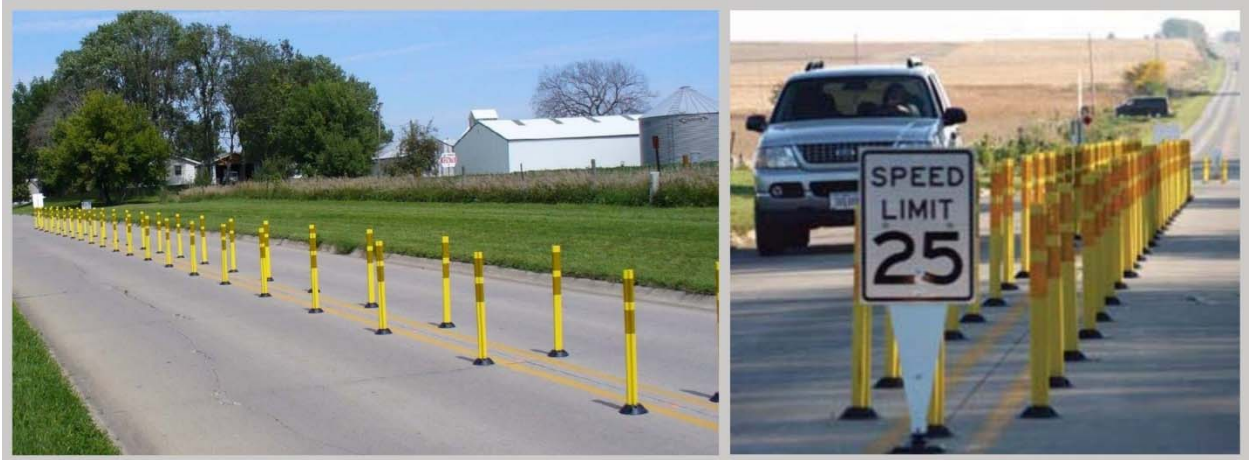
Figure 11 – Sample Channelizer Island
